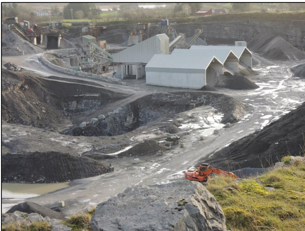
Preparation for further blasting in South Quarry 19 th December 2015.
