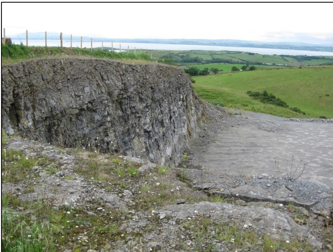
Quarry excavation to west of quarry 2 – looking north- September 2012.
