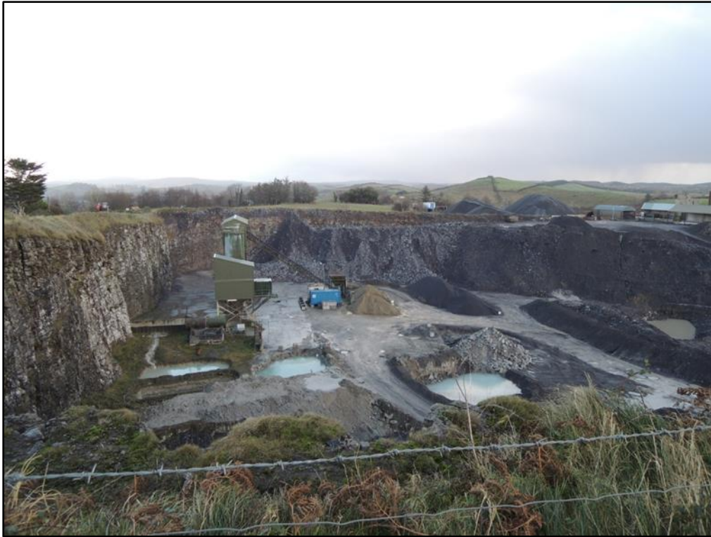
New excavation pits in South Quarry 29 th November 2015.
