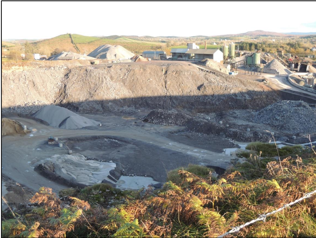
South Quarry new excavation in nase of south quarry floor, October 31 st 2015.
