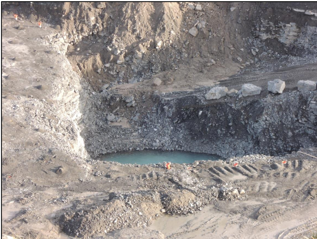
Preparation for further blasting in South Quarry 19 th December 2015 - Blast took place in early January 2016.
