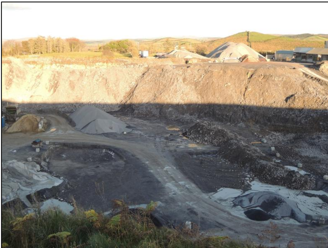
South Quarry new excavation of quarry floor in centre right of photograph 31 st October 2015
